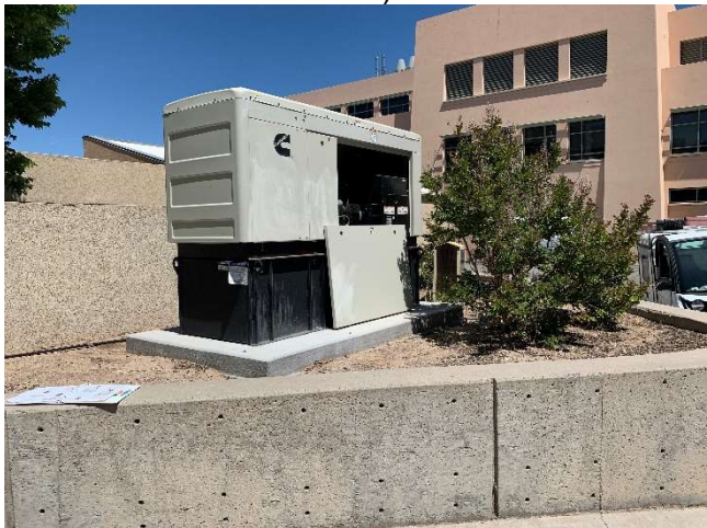
Mechanical Engineering – 122-AST-1 132-gallon diesel emergency generator tank (25 May 2022).
