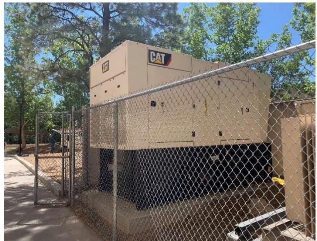
Popejoy Hall – 62-AST-1, 660-gallon diesel emergency generator tank (photo dated 24 May 2022).
