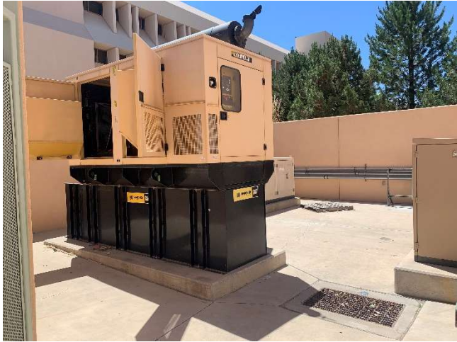
Centennial Engineering Center – 112-AST-1, 660-gallon emergency generator tank (25 May 2022).
