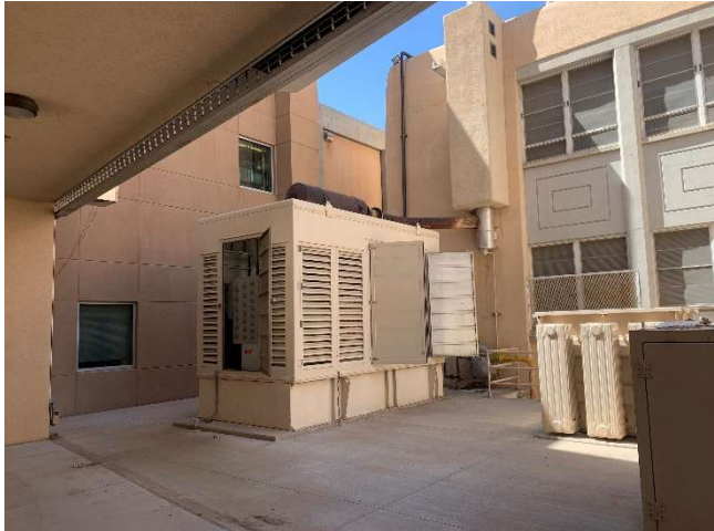
Castetter Hall – 21-AST-1, 1,075-gallon diesel emergency generator tank (24 May 2022).
