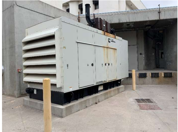
Innovation Discovery Training Complex – 289-AST-1, 500-gallon emergency generator tank (24 May 2022).
