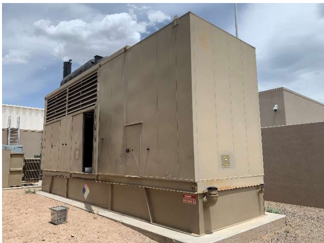
The Pit (University Arena) – 302-AST-1, 2,635-gallon emergency generator tank (23 May 2022)
