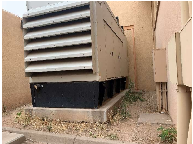
Information Technologies Building – 153-AST-1, 850-gallon diesel emergency generator tank (25 May 2022).
