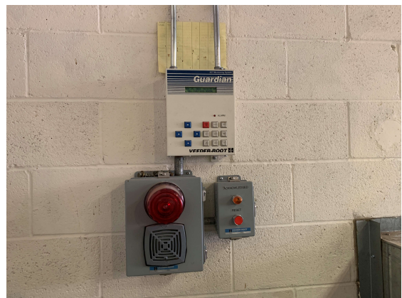
Sandia Crest KNME Transmitter – Veeder-Root Automatic Tank Gauge system (photo dated 25 May 2022).
