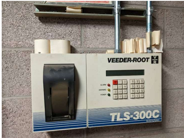
Cancer Research Facility – Veeder-Root Automatic Tank Gauge system (24 May 2022).
