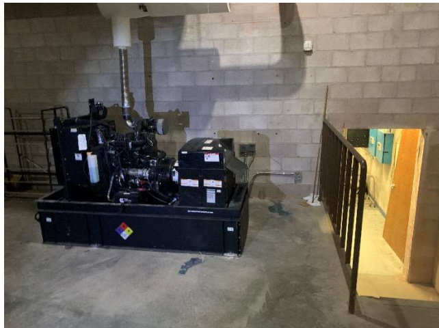
Family Practice Building – 248-AST-1, 76-gallon, emergency generator tank (24 May 2022).
