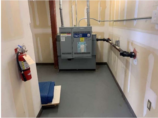
Castetter Hall – Hydraulic Elevator #3: 120-gallon, hydraulic oil reservoir (24 May 2022).
