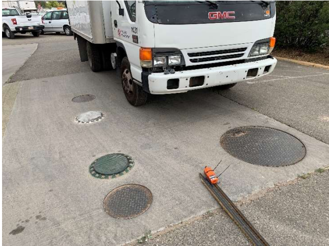
Automotive Center – 216-AST-1A/1B 5,170-gallon vaulted compartment tank (23 May 2022).
