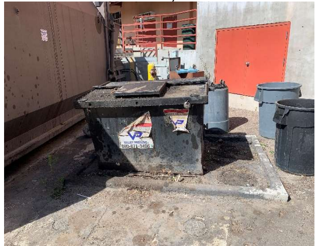
Student Union Building – 60-AST-2 150-gallon cooking grease tank (24 May 2022).
