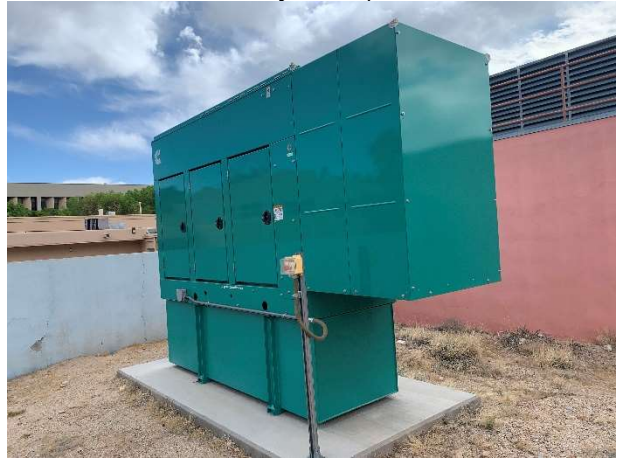
Clinical and Translational Science Center – 227-AST-1, 550-gallon emergency generator tank (24 May 2022).
