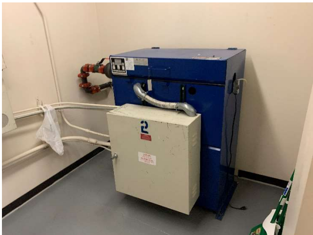
Student Union Building - 120-gallon, hydraulic oil reservoir #2 (24 May 2022).
