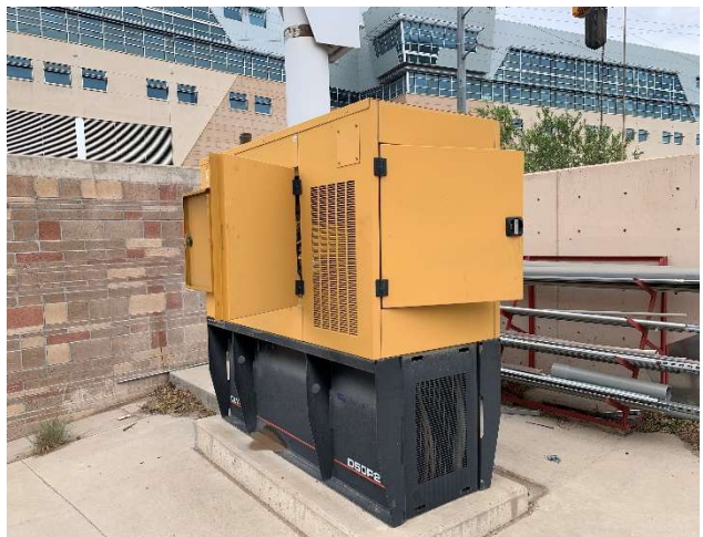
Lomas Chiller Plant – 194-AST-1 147-gallon, emergency generator tank (photo dated 25 May 2022).
