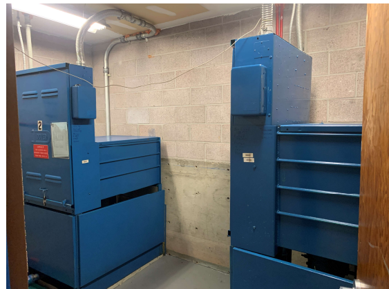
Family Practice Building – Hydraulic elevator machine room with two (2) 120-gallon reservoirs (photo dated 24 May 2022).
