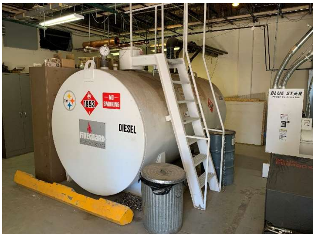
Sandia Crest KNME Transmitter – SC-AST-1, 1,500-gallon, generator supply tank (25 May 2022).
