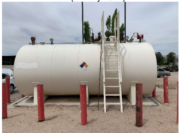
South Golf Course Maintenance Building – 304-AST-1A/1B, 5,000-gallon compartmented supply tank (24 May 2022).
