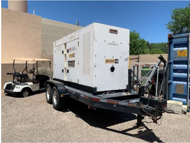
Centennial Sciences and Engineering Library – 46-AST-BACKUP, 79-gallon portable generator tank (24 May 2022).
