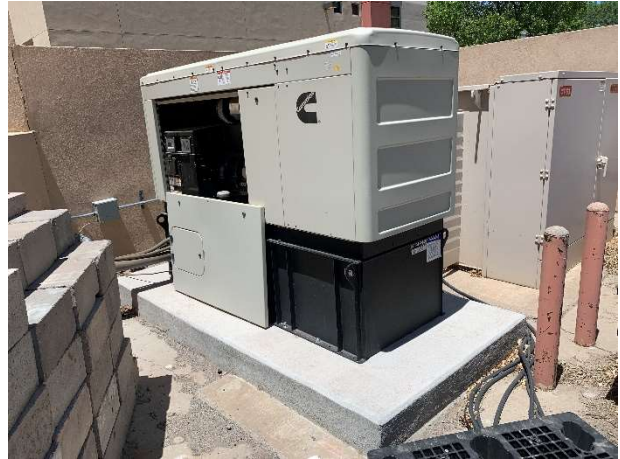
Centennial Sciences and Engineering Library – 46-AST-1, 132-gallon diesel emergency generator tank (24 May 2022).
