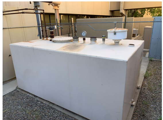
Biological Research Facility and Cancer Research Facility (BRF-CRF) – 229-AST-1, 2,019-gallon diesel supply tank (24 May 2022).
