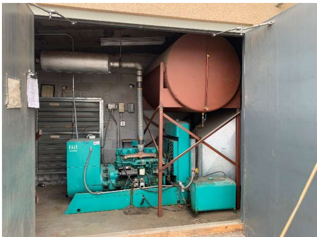
Nursing and Pharmacy – 228-AST-1, 648-gallon, stilted emergency generator tank (23 May 2022).
