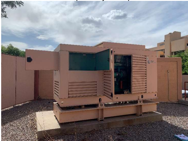
Student Union Building – 60-AST-1 250-gallon diesel emergency generator tank (24 May 2022).
