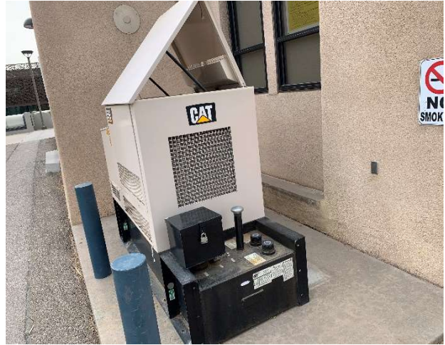
Economics Hall – 57-AST-1, 140-gallon diesel emergency generator tank (24 May 2022).
