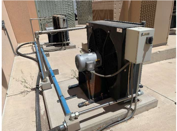
Centennial Engineering Center – 112-AST-1, pump set with audible alarm (25 May 2022).
