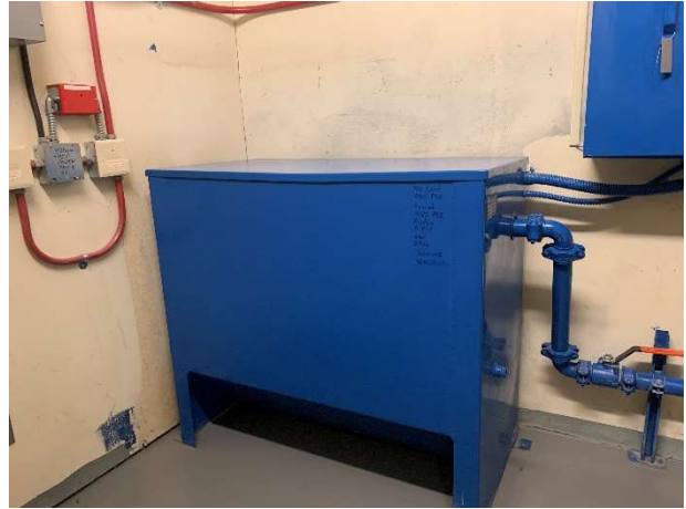
Castetter Hall – Hydraulic Elevator #2: 120-gallon, hydraulic oil reservoir (24 May 2022).
