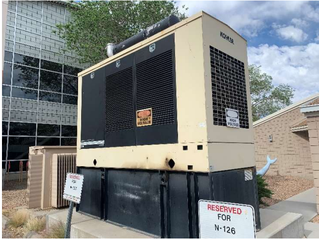
Research Incubator Building – 205-AST-1, 750-gallon emergency generator tank (24 May 2022).
