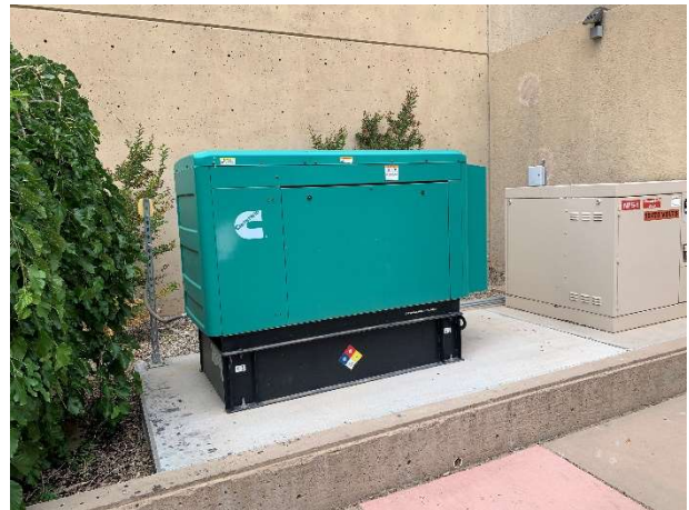
Health Sciences Library and Informatics Center – 234-AST-1, 50-gallon emergency generator tank (24 May 2022).
