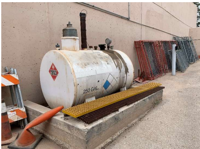
Lomas Chiller Plant – 194-AST-1 250-gallon, waste oil tank (25 May 2022).
